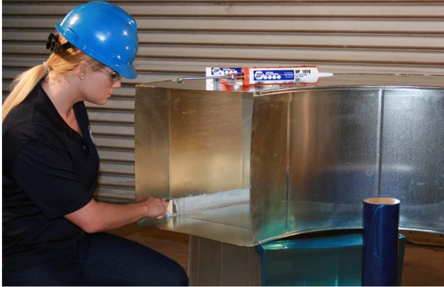
Amanda Baker of Control Air in Anaheim, California, seals duct.
