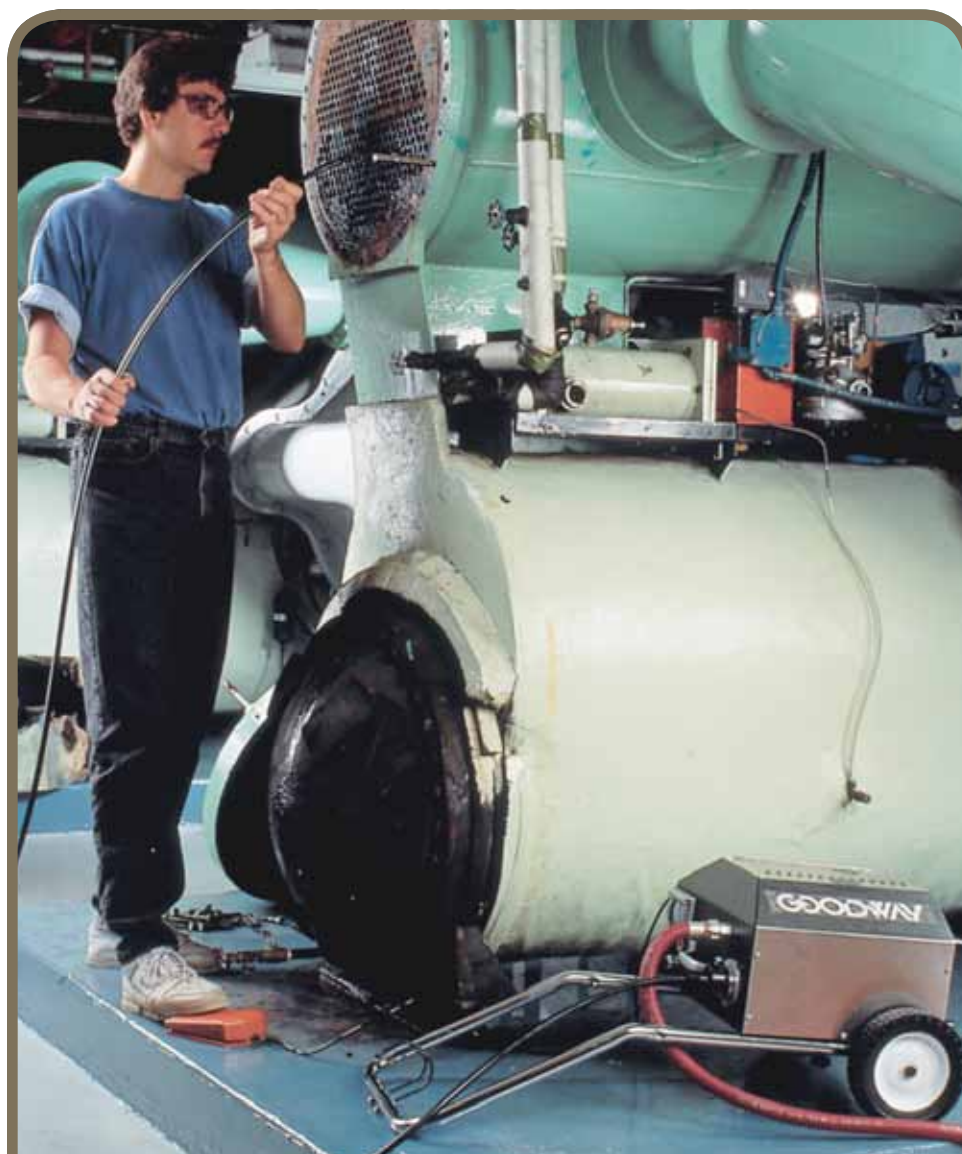
Figure 3 (left). The man above is cleaning the condenser tubes on a large chiller using a machine that turns a nylon brush and flushes the tube with water at the same time. (©Delmar Cengage Learning.)
