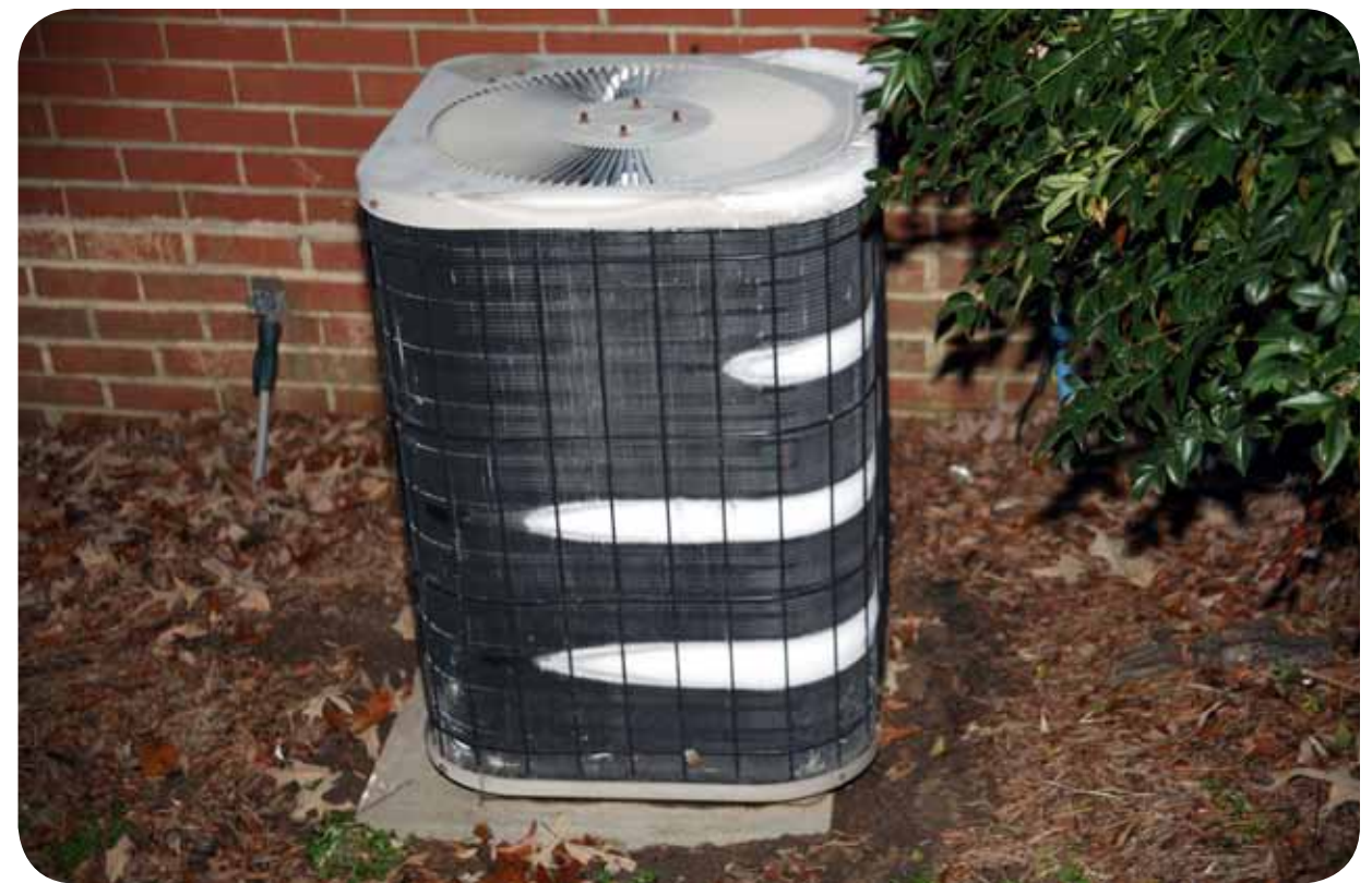
Figure 1. This frosted heat pump does not have enough refrigerant. You can see the various refrigerant circuits in the coils. (Photo by Bill Johnson)
