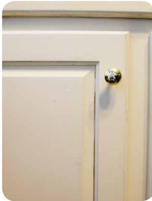
Figure 1 (left). This is a photo of a cabinet door that is showing shrinkage due to low humidity. (Photo by Bill Johnson) Figure 2 (above). A sling psychrometer uses the wet-bulb/dry-bulb principle to provide humidity readings. (From Refrigeration & Air Conditioning Technology, 5th Edition, by William Whitman, William Johnson, and John Tomczyk, published by Delmar Cengage Learning.) (©Delmar Cengage Learning.)
