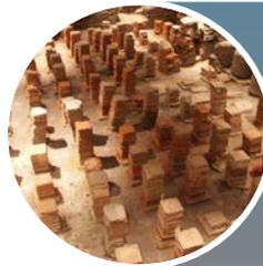
The Greeks and Romans began using hypocausts, which featured floors raised up on pillars as hot air passed in the space beneath.
