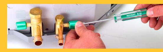
Seal service valve to prevent leaks
