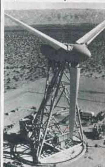
STANDING 20 STORIES HIGH, this giant windmill will generate 6 million kWh this year, the energy equivalent of about 10,000 barrels of fuel oil. It converts wind energy into electricity for as many as 1,000 homeowner customers of Southern California Edison Co. The Louis Allis synchronous alternator which converts the rotating energy into usable power was produced at the company's Beloit, Wis., facility.
