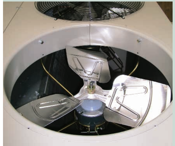
Totally enclosed fan motors prevent electrical damage from rain and condensation.
