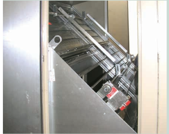
Standard low-leak dampers provide superior leakage rates per ASHRAE Standard 90.1-2004.
