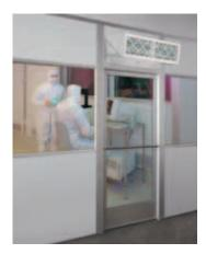
The Mars **Hepac** Air Curtain, featuring H.E.P.A. (High Efficiency Particulate Air) filters, effectively removes airborne contaminants to meet even the most rigid military, federal and health standards. This gentle moving air barrier provides a downflow curtain of ultra-clean air when installed over open doorways isolating your outside contaminated areas while it filters air inside the room for double protection.
