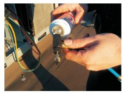
air temperature down to the dew point where micro droplets of water are deposited around the perimeter of the leak area. When the sealant comes in contact with the droplets of water it begins to form a permanent low tensile crystalline structure, which creates a barrier preventing the refrigerant from escaping.
