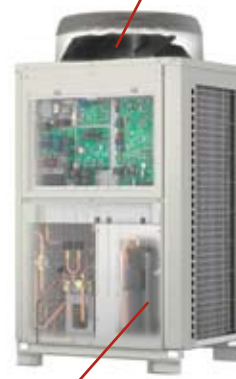
High performance R410A INVERTER-driven scroll compressor
